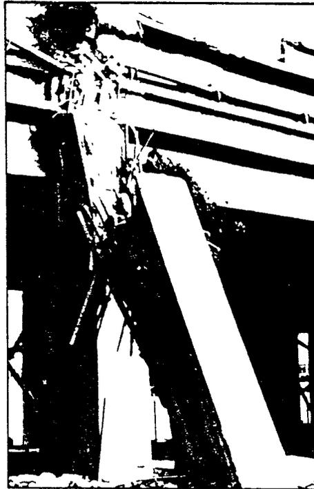
Figure 1.11 Failure of the West Side of Bent 90
