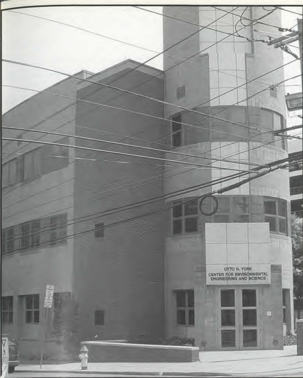
The York Center for Environmental Engineering and Science is the home of many of NJIT's environmental programs and initiatives.
