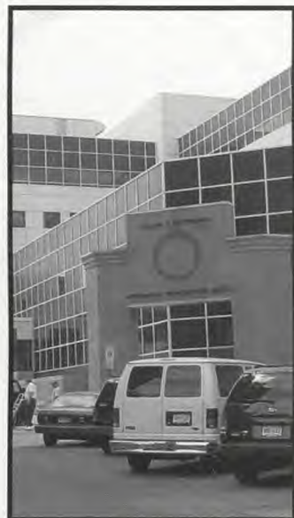
The five-story, $30 million Guttenberg Information Technologies Center was designed to provide state-of-the-art facilities for education and research in manufacturing, robotics, information technology and telecommunications.
