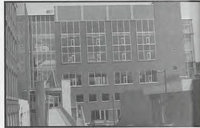
Summit Street side of the School of Architecture building, Weston Hall.
