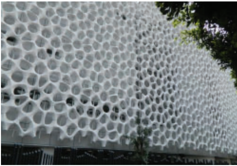
Air Filtering Facade System Manuel Gea Gonzalez Hospital, Mexico City
