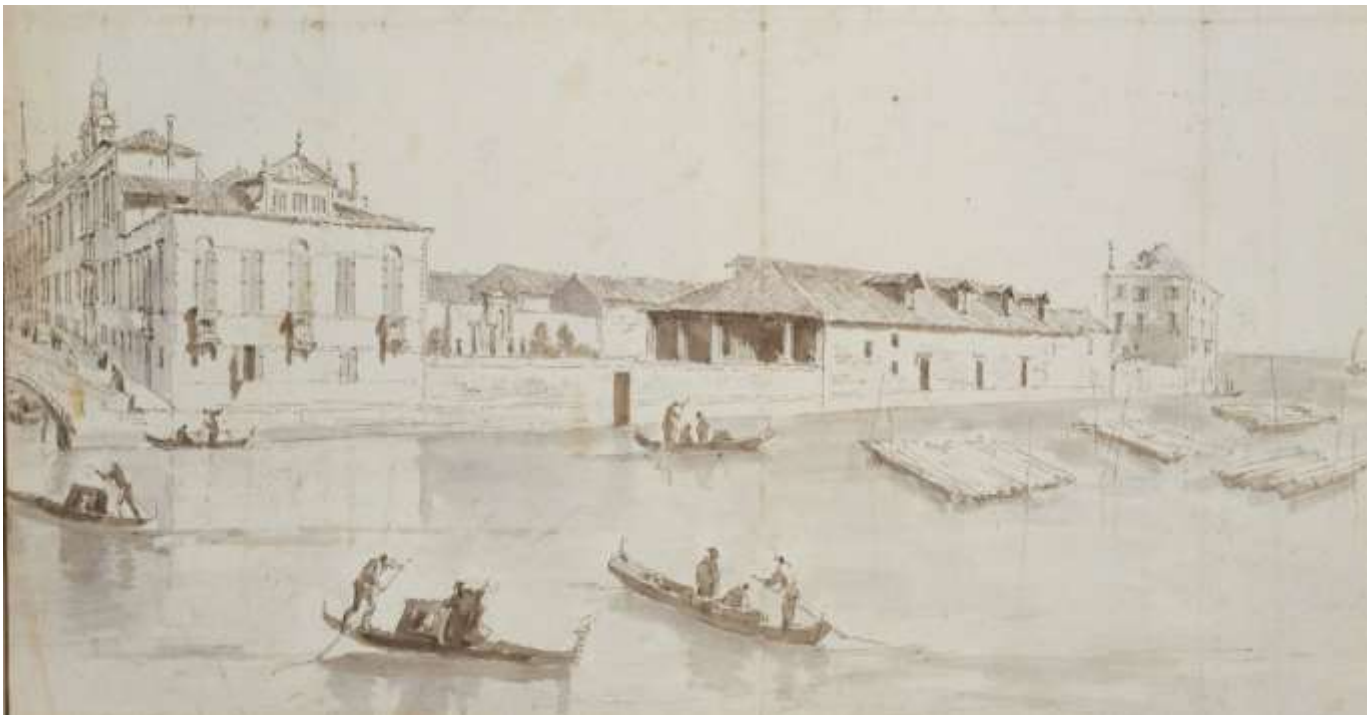
Historical view of western site boundary.
