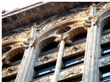
Louis Sullivan, Bayard Building, New York, façade detail
