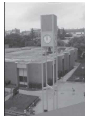
CHRISTINA CROVETTO The clock tower and carillon sit in a European-style plaza adjacent to the newly-renovated Campus Center.
